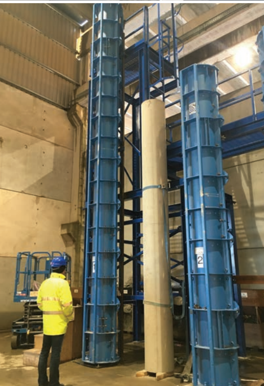
Above: Bespoke column moulds at Banagher Precast Concrete.
