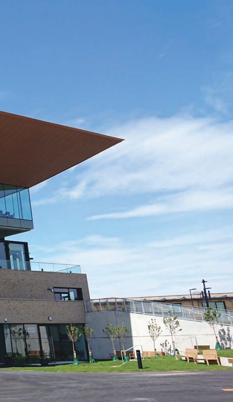
Completed 'Aga Khan' grandstand with iconic roof.
