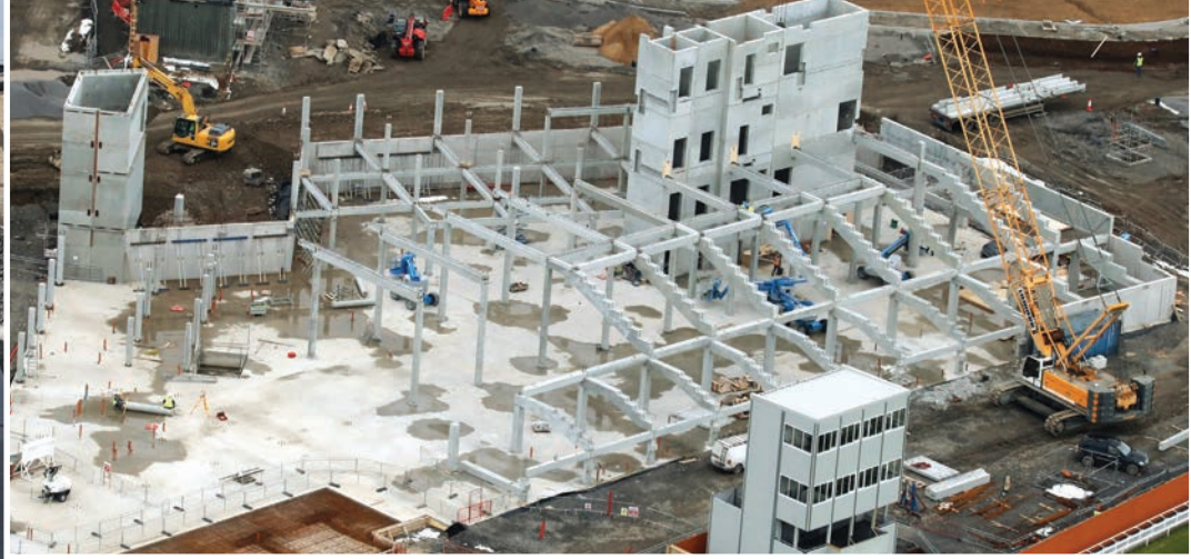
Precast installation on-site.
