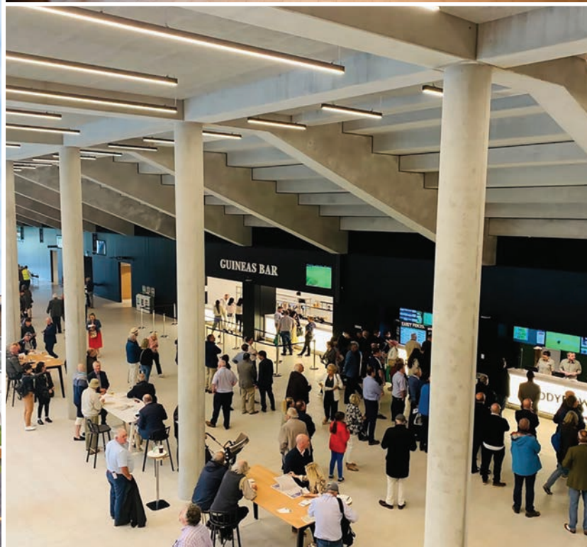
Champions Hall, showing raker beams and terrace units.
